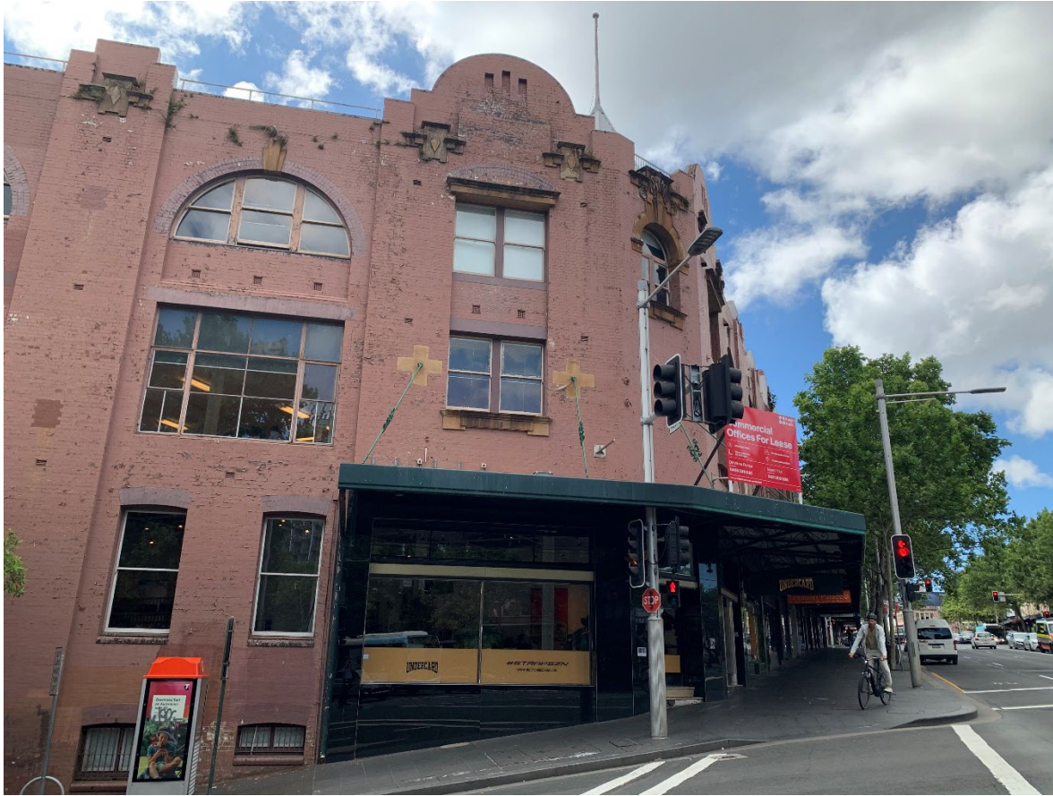
Group 2 viewed from the western side of Crown Street
